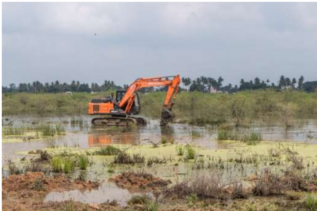
Figure 2 Diggers clearing earth and vegetation from the wetland
